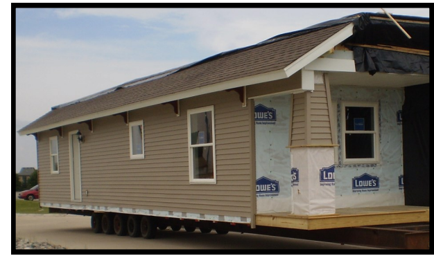
Above: House built for Macomb County Habitat for Humanity in 2016. Fabricated inside the Construction Trades building at Dakota HS, the house is built in two halves and transported to its permanent site.
